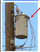
This is a typical step-down transformers used to bring the line voltage down from 5000 V to 240 V before it gets to your home
